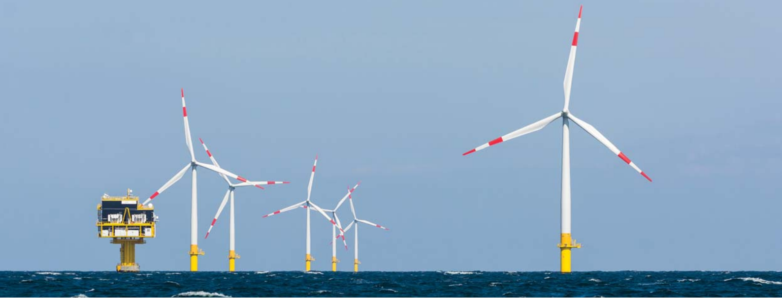
Topside offshore converter station and wind turbines.
