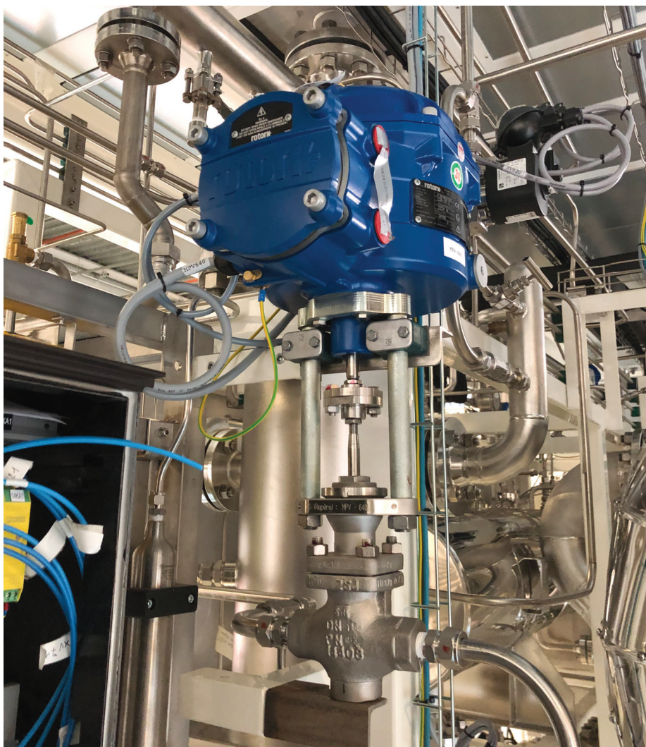
Rotork is also active in the green hydrogen market, supplying CVL-500 actuators to companies such as AREVA H 2 GEN.
