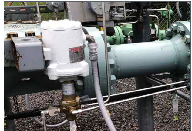
PAX 1 installed in pressure control and metering stations for natural gas distribution
