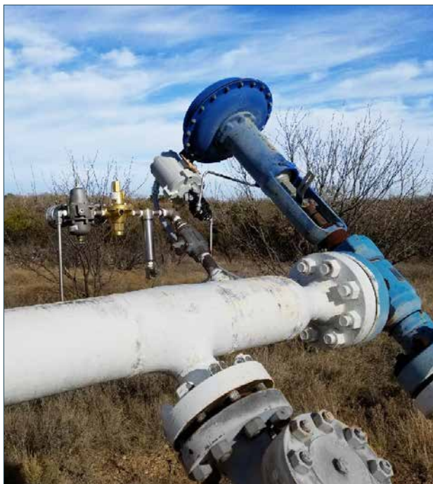
PAX 1 installed on natural gas pipeline, as a pilot for the Control Valve
