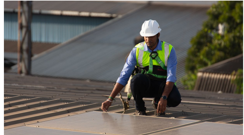
We installed solar panels at our Gimpo (South Korea) facility in 2023
