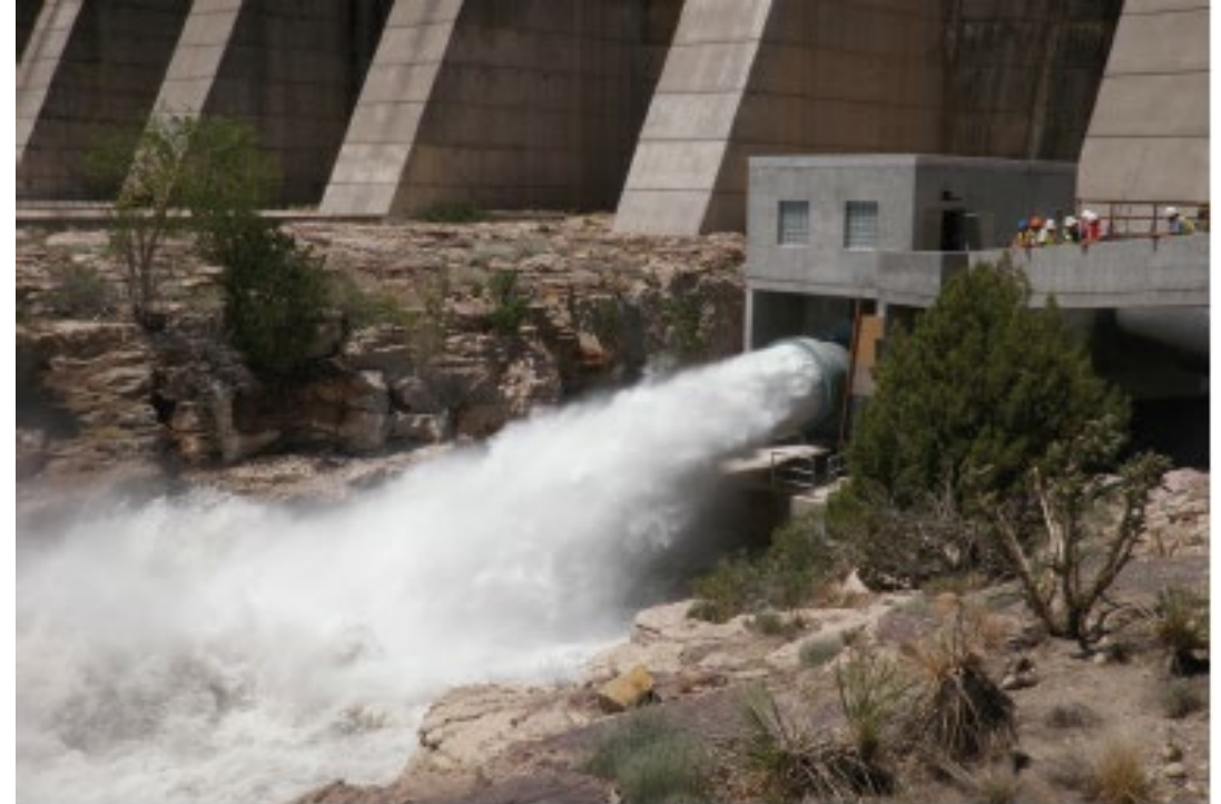
The Pueblo dam in Colorado, USA, in operation with reservoir water flowing through a 60-inch valve of the type shown on the left (complete with Rotork IQ actuator) © Howell Bunger
