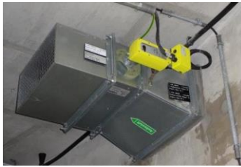
Damper on Ventilation System in Biogas Reactor
