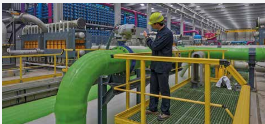
Water treatment plant in Spain
