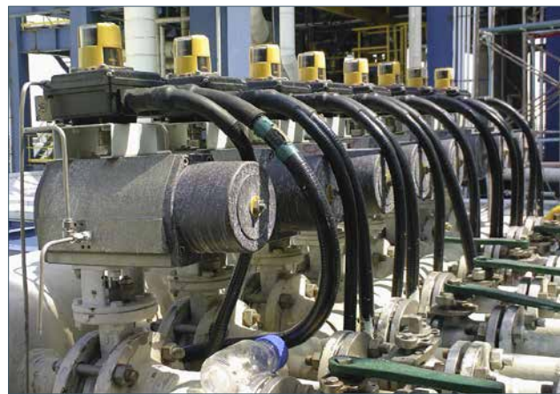
For reference: older installed RCT actuators
