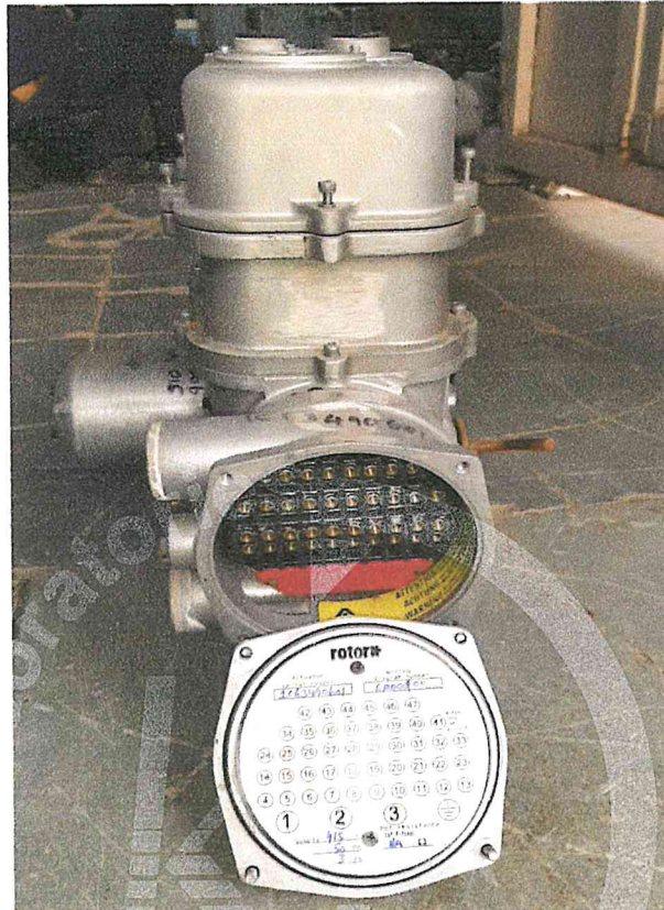
Pictute3: No ingress of powder & water observed
