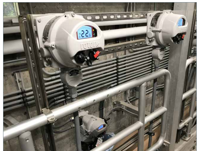
RHS Pro operating IQT3 Pro actuator in an inaccessible location
