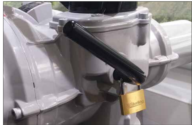
Fig 7.1. IQ3 hand-auto lever padlocked
