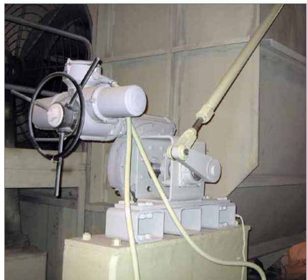
IQ Series on ID Fan Inlet Damper
