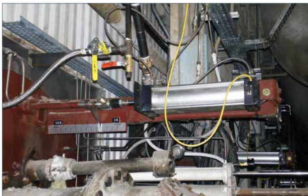
JR Series wall-fired burner shroud
