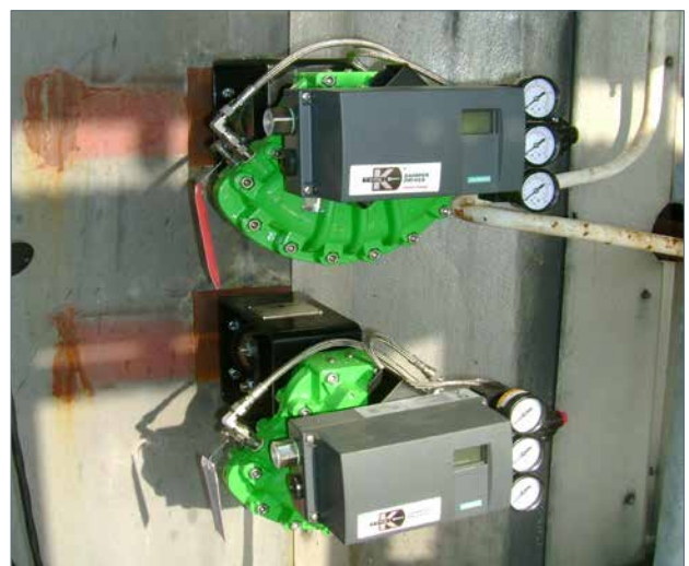
TYPE K DM Series on Windbox application
