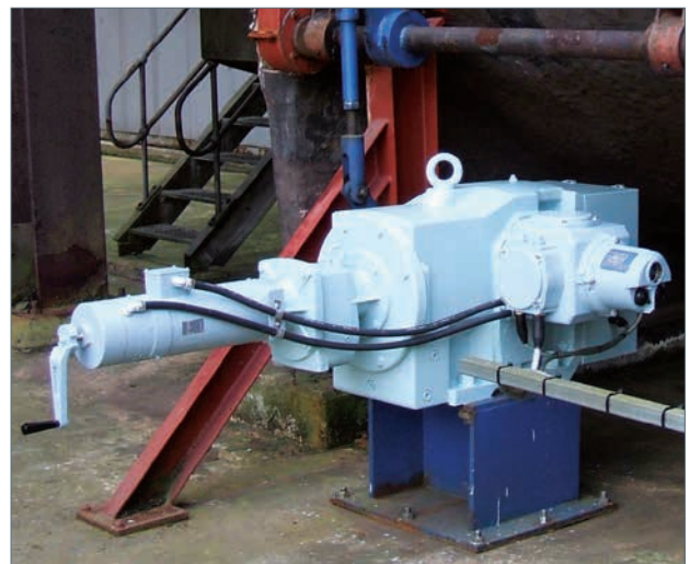
SM-6000 Series on Induced Air Fan Damper
