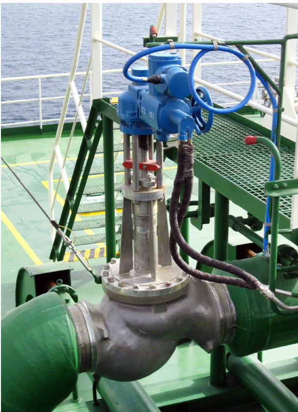
Figure 2. Rotork 4H multi-turn actuators mounted on a cryogenic globe valve on an LNG carrier.
